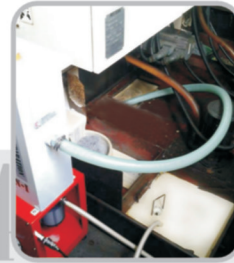
4 Place outlet pipe on CNC water tank(Keep free flowing).
